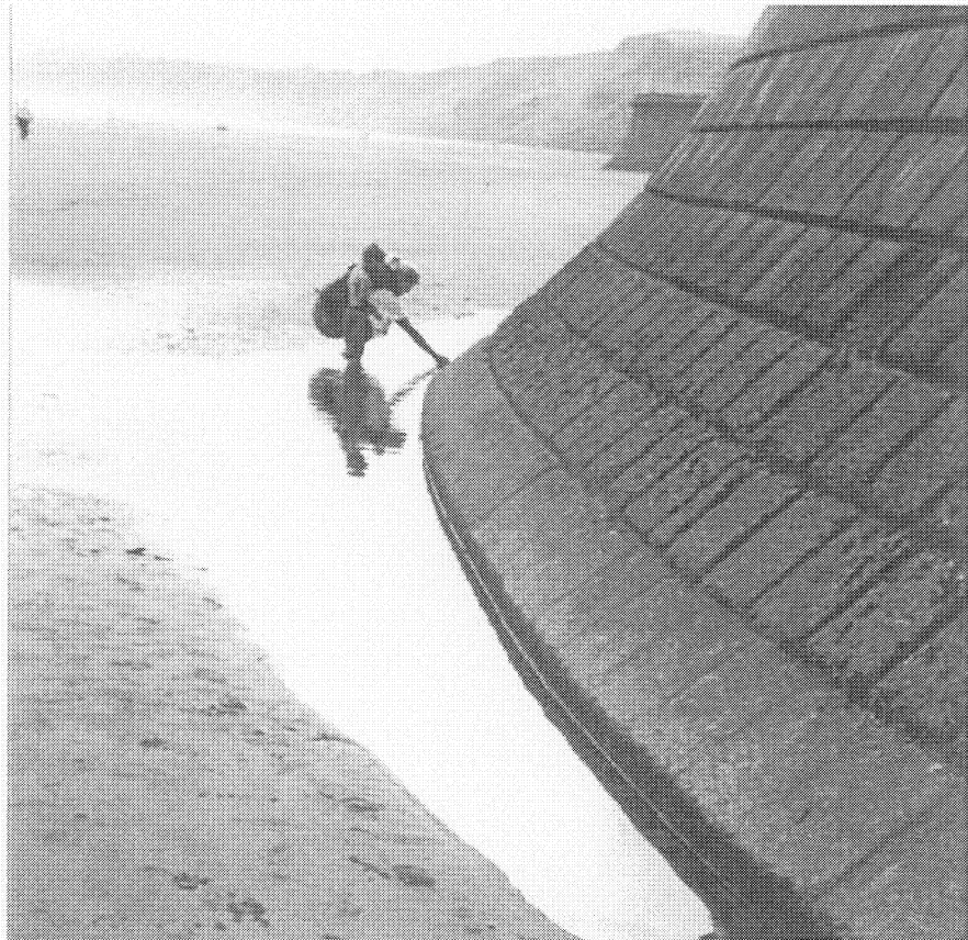
Figure 7.4 Scour at base of Filey seawall
