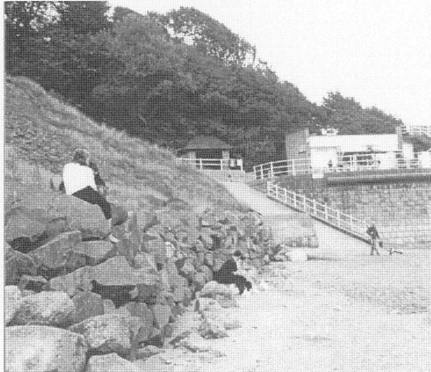
Figure 7.3 Rock protection adjacent to Martin's Ravine to south of Filey Town
